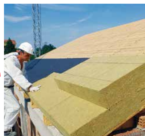
PITCHED ROOFS THERMAL INSULATION ABOVE THE RAFTERS
